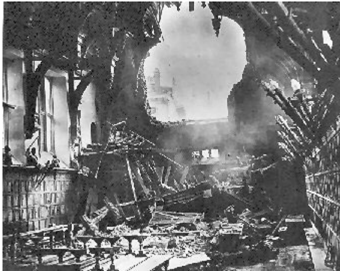
Damage to the Screen, World War II
